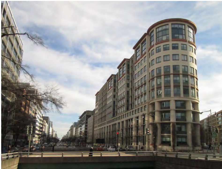
4 22ND STREET LOOKING EAST DOWN K STREET
