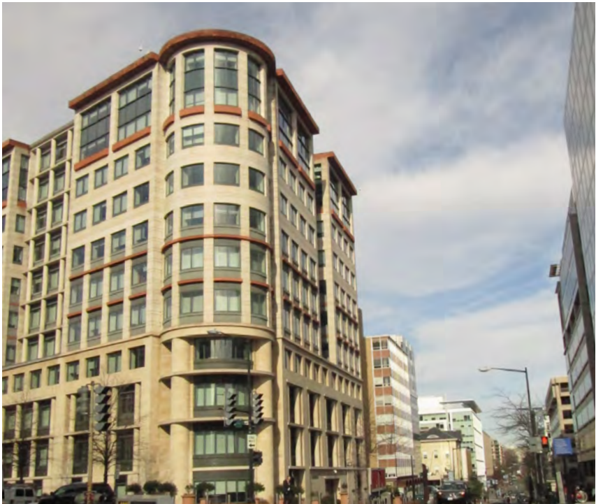
3 PENNSYLVANIA AVE. LOOKING NORTH DOWN 21ST STREET
