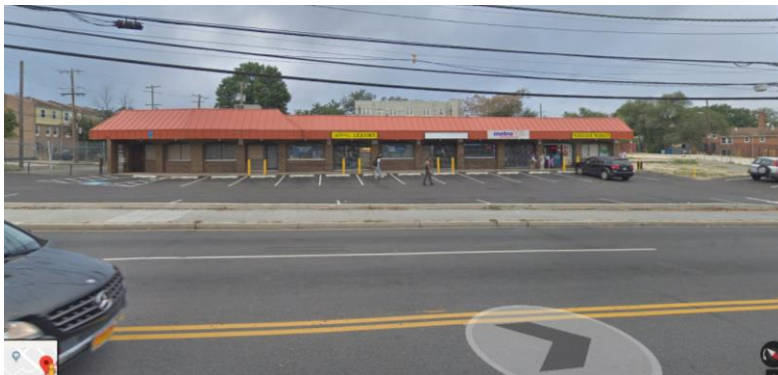
Existing Site Condition (2019)
