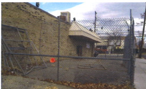
AT REAR ALLEY / SIDE RETAIL LOOKING TOWARDS WHEELER ROAD
