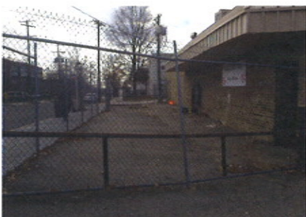
CORNER WHEELER ROAD & BARNABY STREET LOOKING TOWARD RETAIL REAR ALLEY
