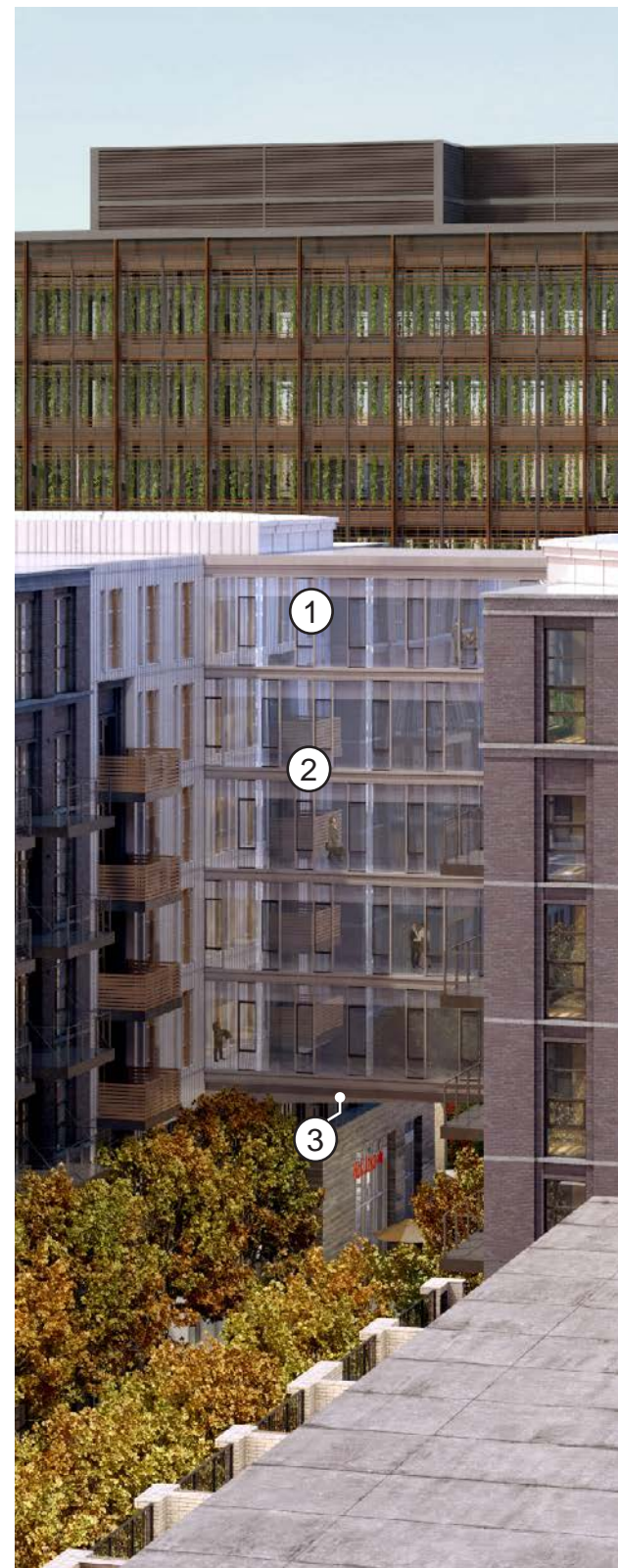
PARTIAL VIEW FROM SOUTHEAST
