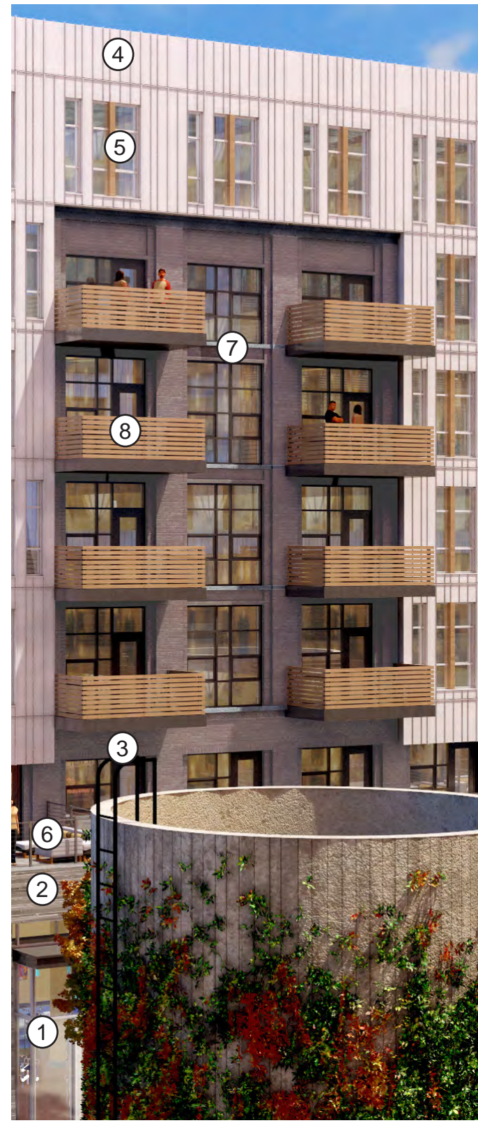
PARTIAL VIEW FROM NORTH
