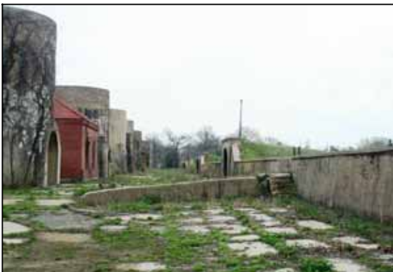
Service Court, 2008 (EHT Tracerics, Inc.)
