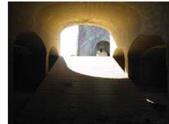
Filter bed ramp, existing condition
