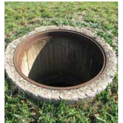
Manhole opening, existing condition
