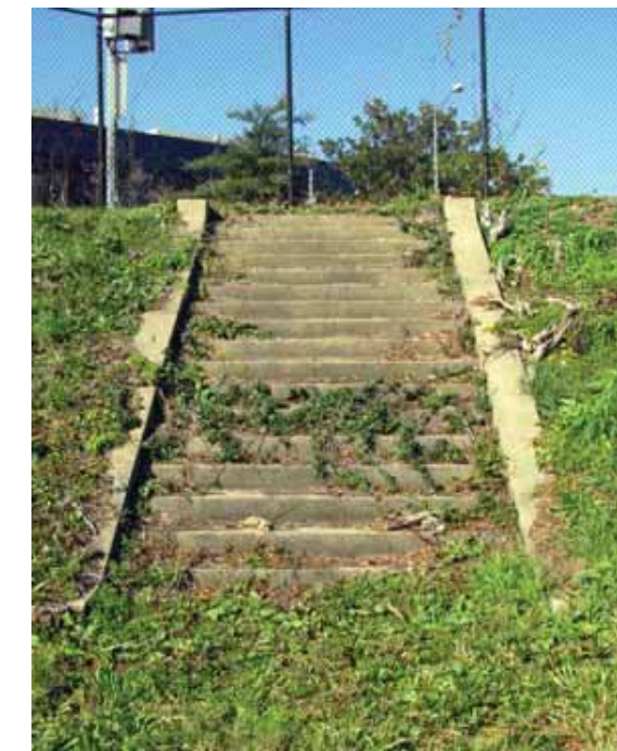
Corner stair, existing condition
