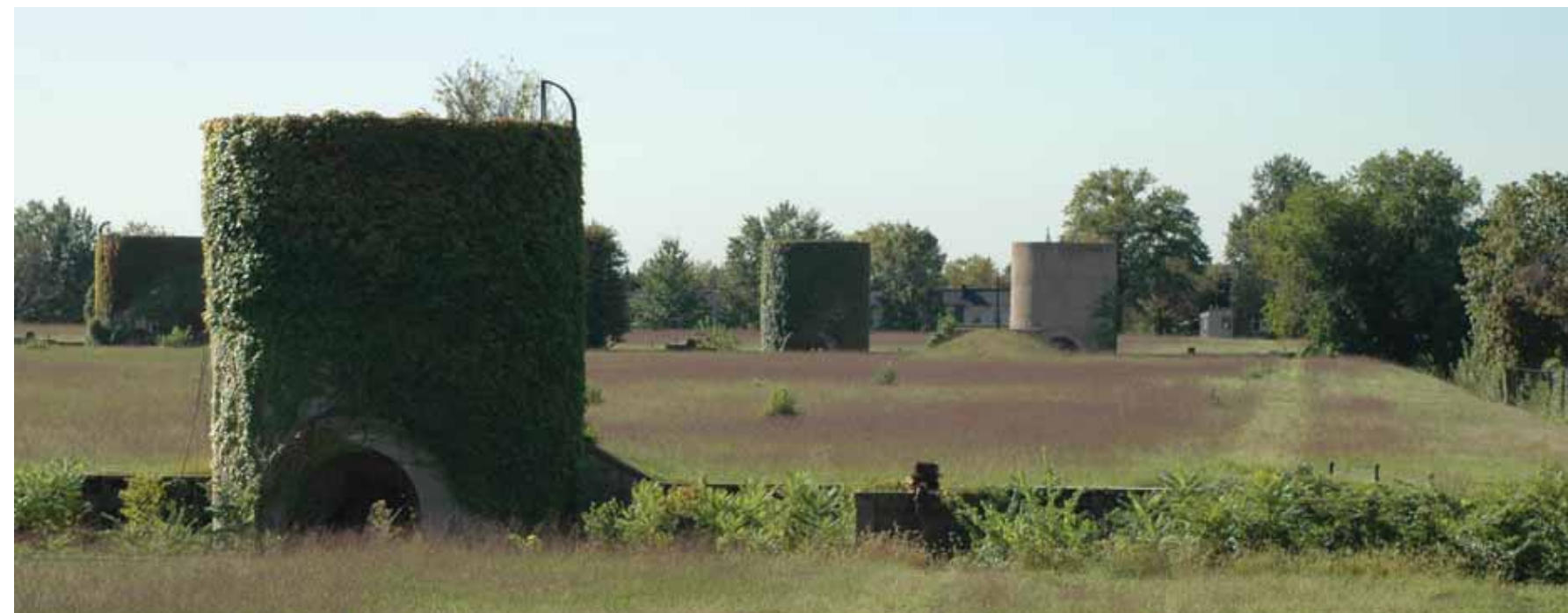
McMillan Site, existing condition
