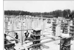
FILTRATION PLANT SHOWN DURING CONSTRUCTION
