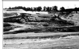
FILTRATION PLANT SHOWN DURING EXCAVATION
