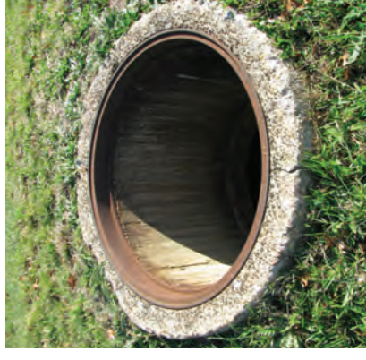
Manhole opening, existing condition
