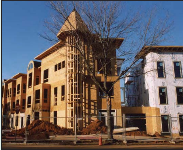
Kentucky Courts Redevelopment
