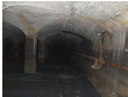
FIG. B.7 - HINGE FORMATIONS ALONG THE END WALLS AND BETWEEN PIERS.
