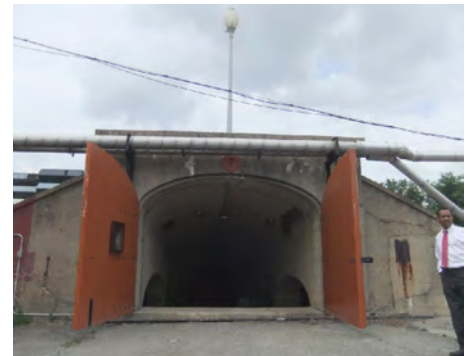
FIG. B.2 - ENTRANCE TO FILTER No. 7.
