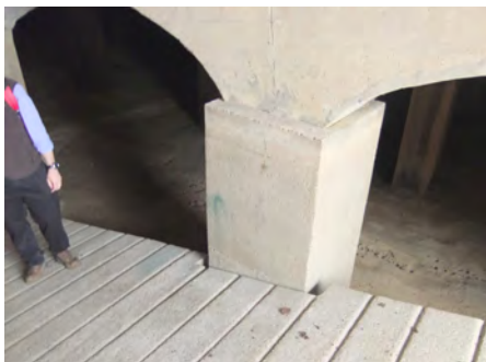
FIG. B.8 - RETROFIT TO COLUMNS AT THE ENTRANCE RAMP.
