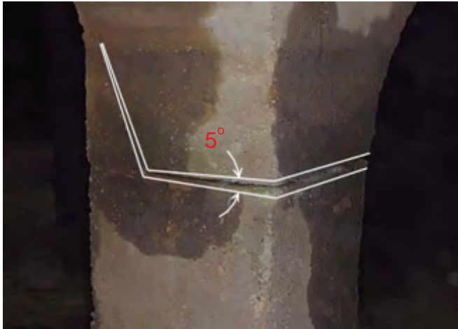
FIG. C.5 - TYPICAL ROTATION AT ENTRANCE RAMP PIER-TO-CEILING JOINT.
