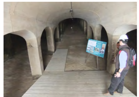
FIG. B.3 - FILTER No. 7 BOARDWALK AND FILTRATION PROCESS DISPLAY.
