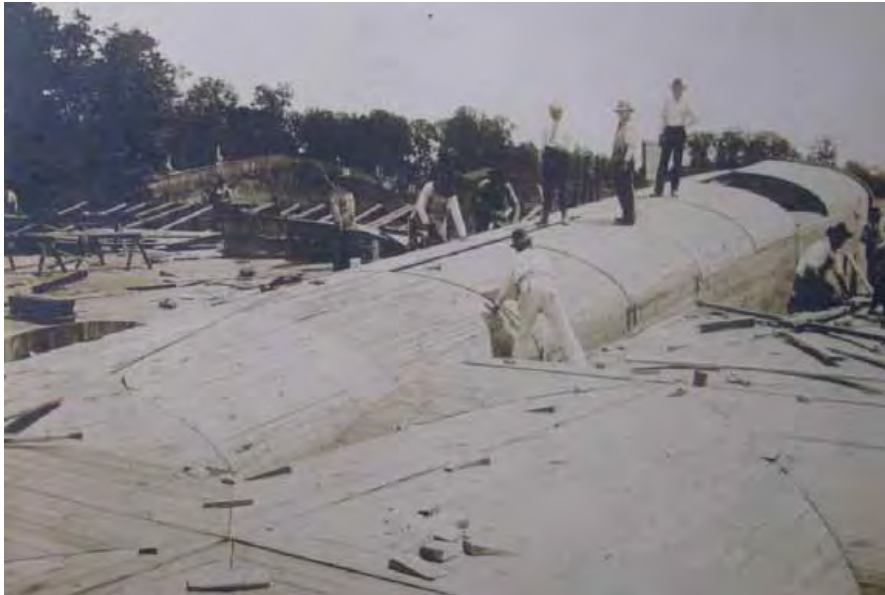
FIGURE 4: PHOTO SHOWING TOP SIDE OF FORMWORK OF TYPICAL BAY IN FOREGROUND AND ENTRANCE RAMP BEYOND (1902-1904), COURTESY OF THE ARCHIVES OF THE WASHINGTON AQUEDUCT
