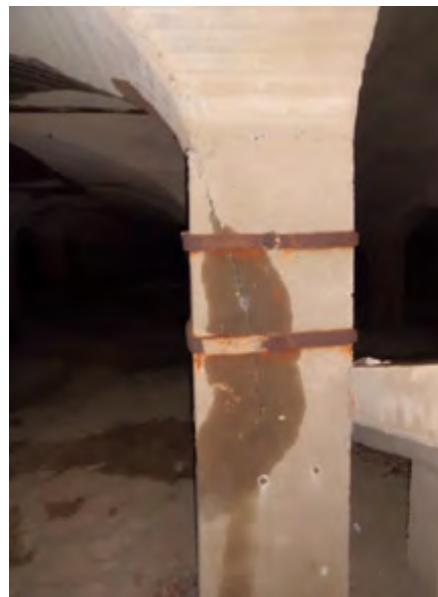
FIGURE 13: PORTAL ENTRANCE PIER AT SLOW SAND FILTER No. 26
