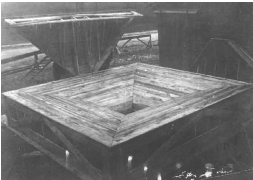
FIGURE 4: PHOTO SHOWING TOP SIDE OF FORMWORK OF TYPICAL BAY IN FOREGROUND AND ENTRANCE RAMP BEYOND (1902-1904), COURTESY OF THE ARCHIVES OF THE WASHINGTON AQUEDUCT
