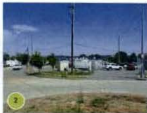
M STREET WEST ENTRANCE
