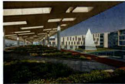
ROOF OVERHANG WITH SKYLIGHTS
