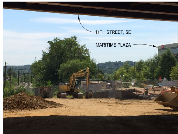
VIEW SOUTHEAST FROM UNDER 11TH STREET BRIDGE ⑥
