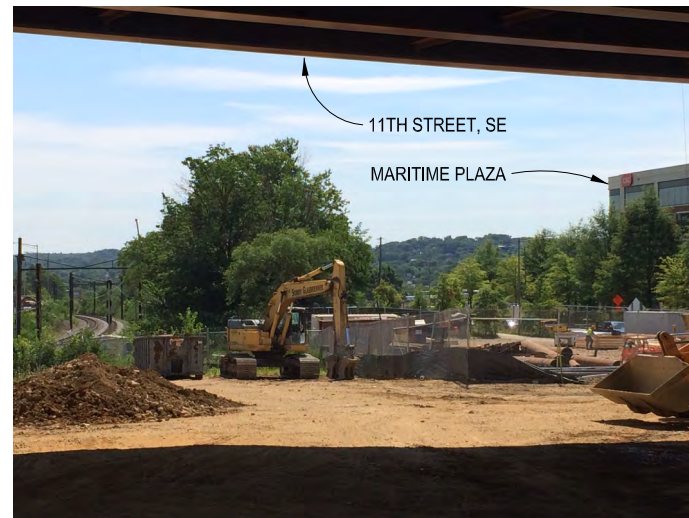
VIEW SOUTHEAST FROM UNDER 11TH STREET BRIDGE 6
