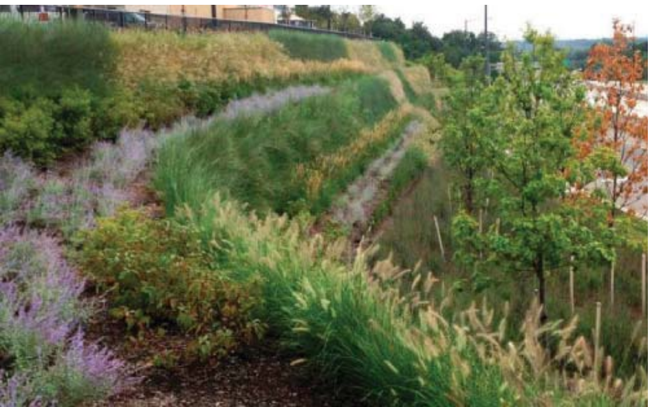
Smart slope - vegetated retaining wall
