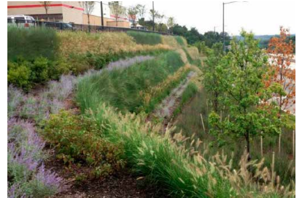
Smart slope - vegetated retaining wall
