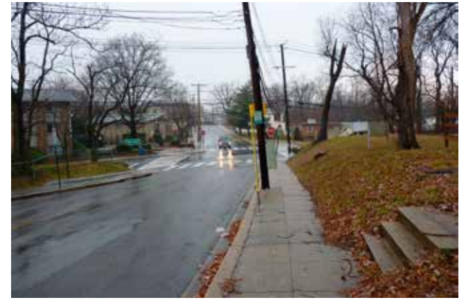
5 - View SE on Elvans Road Road
