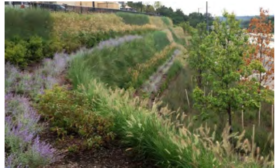
Smart slope - vegetated retaining wall
