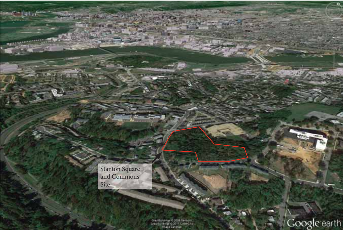
Aerial View of Site and Context
