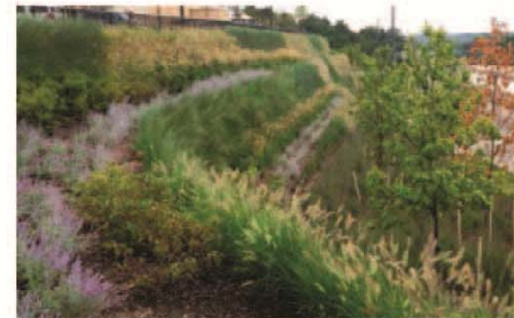
Smart slope - vegetated retaining wall
