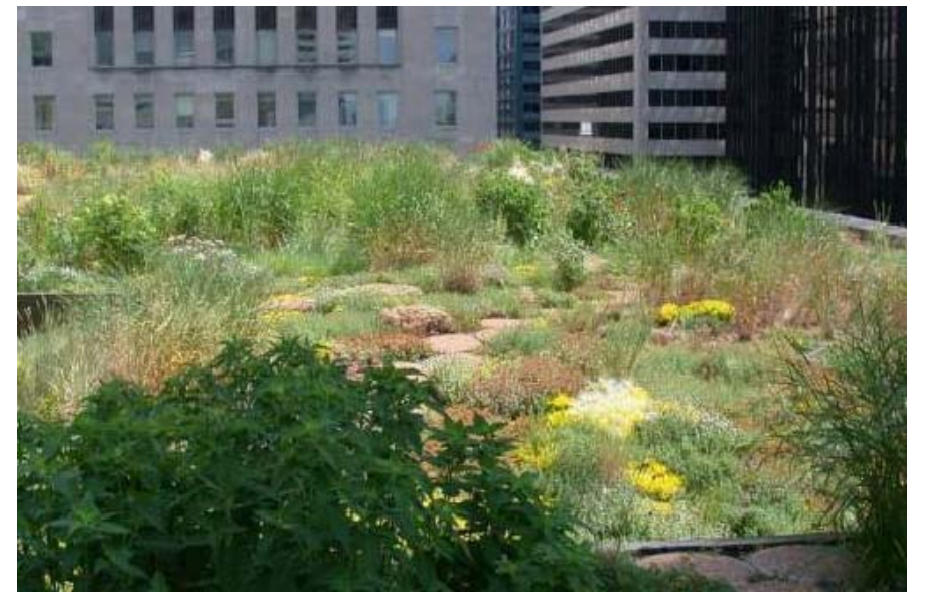
INTENSIVE GREEN ROOF PLANTINGS
