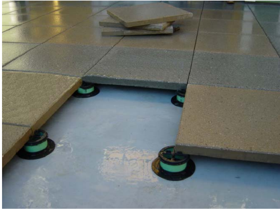
PRECAST CONCRETE PAVERS ON PEDESTAL
