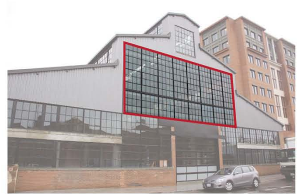
EXISTING BOILER MAKER BUILDING
