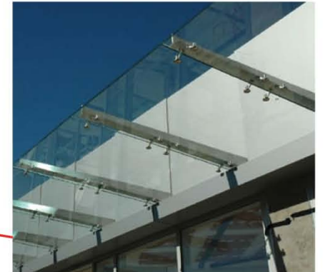
Glass Canopy held with Spider-Fitting Ribs
