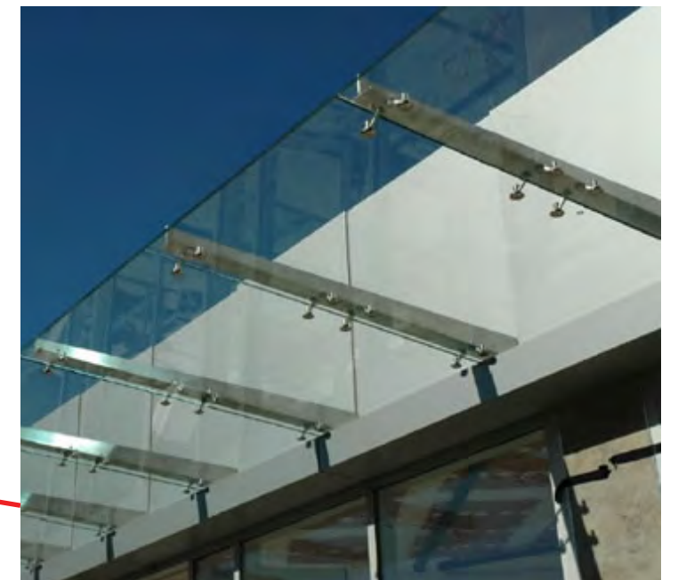
Glass Canopy held with Spider-Fitting Ribs
