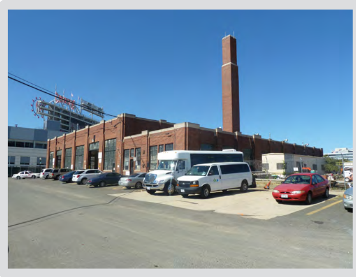
EXISTING IMAGES FLEET MAINTENANCE BUILDING
