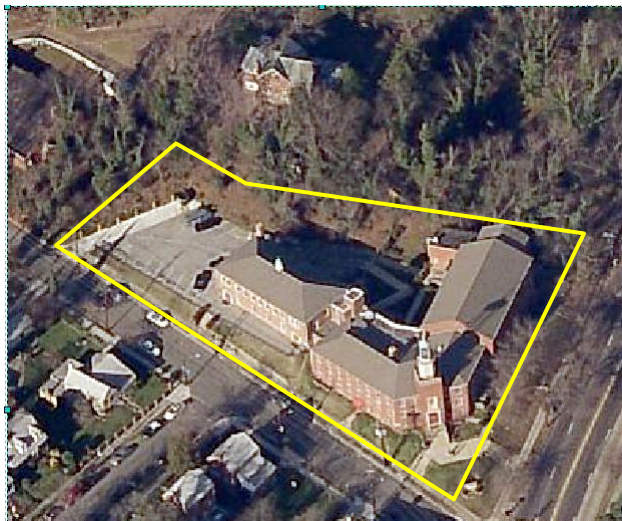
Current Photograph of Site
