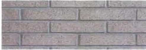
BRICK 1 - EAST BUILDING AND SAWTOOTH BAYS
