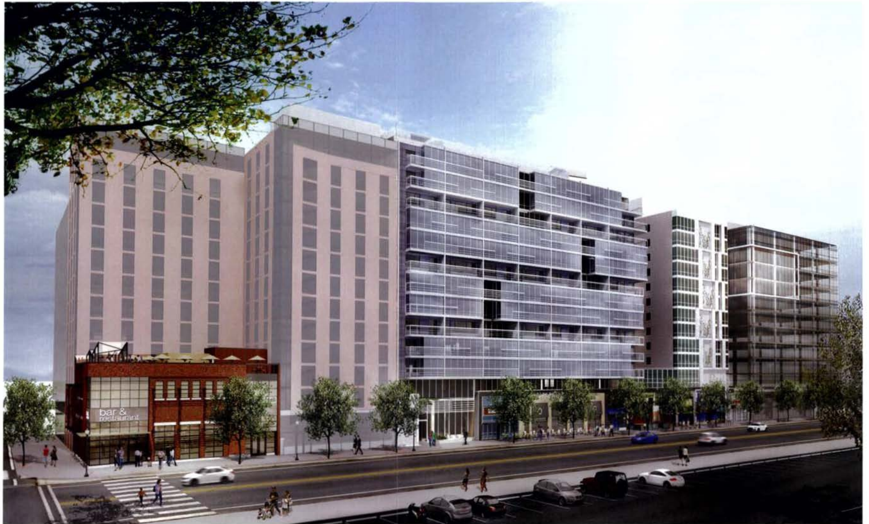
VIEW OF FIRST STREET SE
