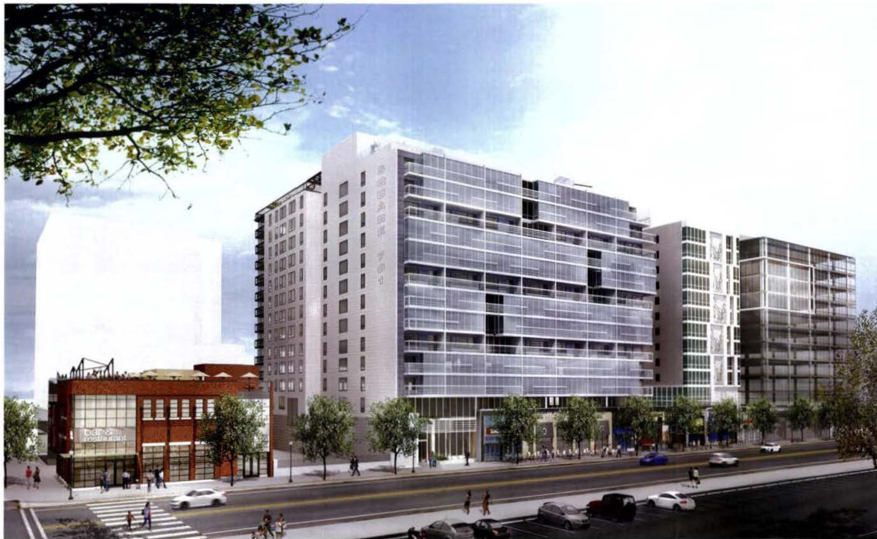
VIEW OF FIRST STREET SE
