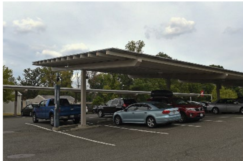
Solar canopy at O'Boyle Parking Lot
