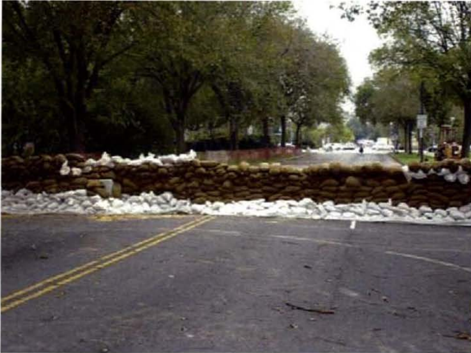
Sandbag closure on 17th Street, NW
