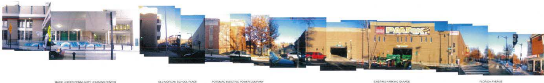
2 T-1.2 EXISTING PHOTO CHAMPLAIN STREET ELEVATION (LOOKING EAST) N.T.S.
