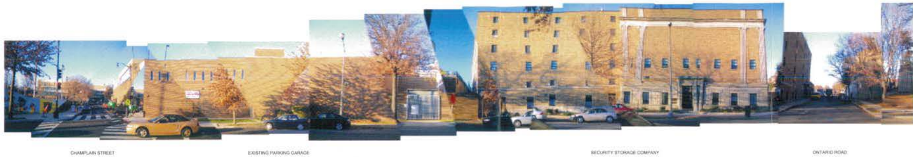
1 T-1.2 EXISTING PHOTO FLORIDA AVENUE ELEVATION (LOOKING NORTH) N.T.S.
