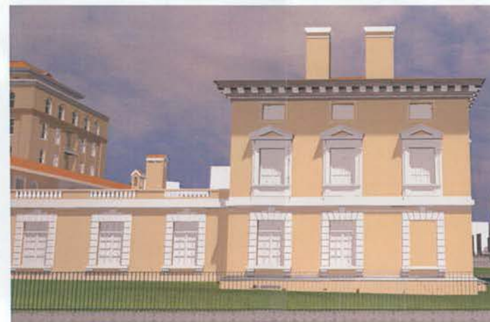
VIEW OF WINDOW RESTORATION
