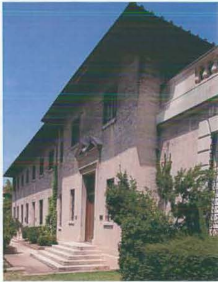
VIEW OF EXISTING CHANCERY
