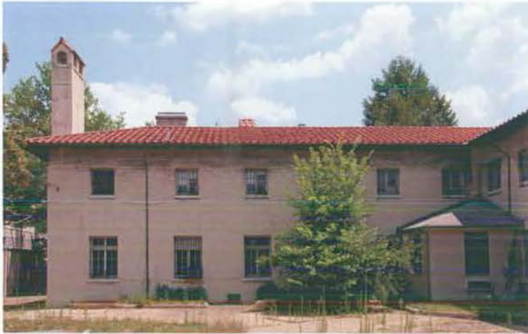
EXISTING CHANCERY WING ROOF
