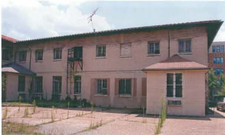
EXISTING CHANCERY WING WINDOWS
