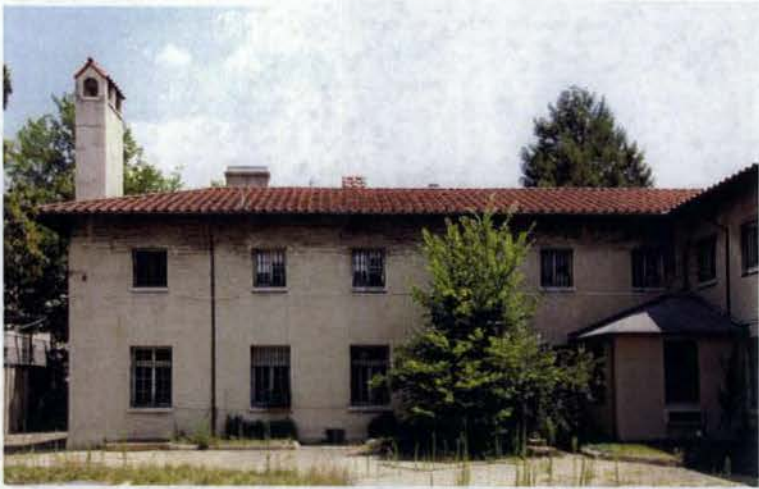
EXISTING CHANCERY WING ROOF
