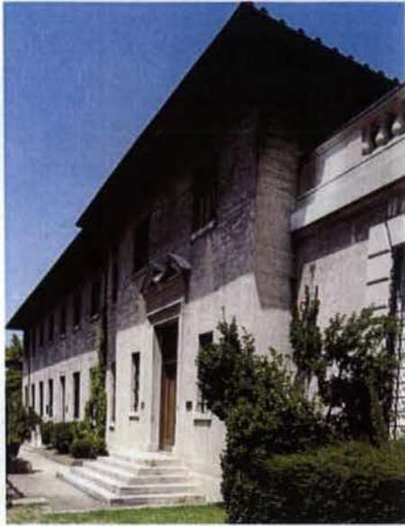
VIEW OF EXISTING CHANCERY
