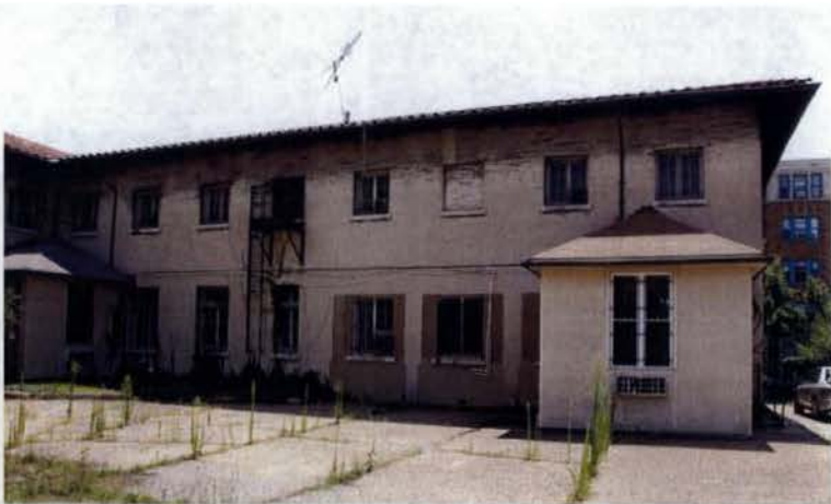
EXISTING CHANCERY WING WINDOWS
