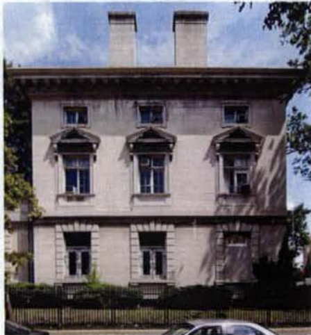
VIEW OF EXISTING WINDOWS
