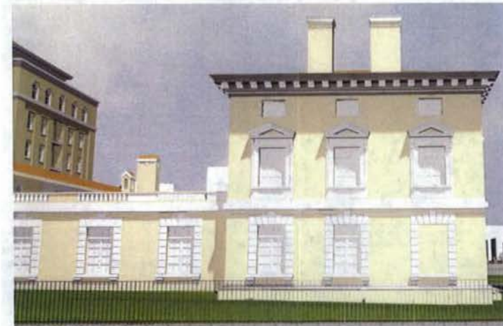
VIEW OF WINDOW RESTORATION
