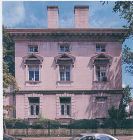
VIEW OF EXISTING WINDOWS
