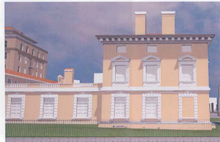
VIEW OF WINDOW RESTORATION
