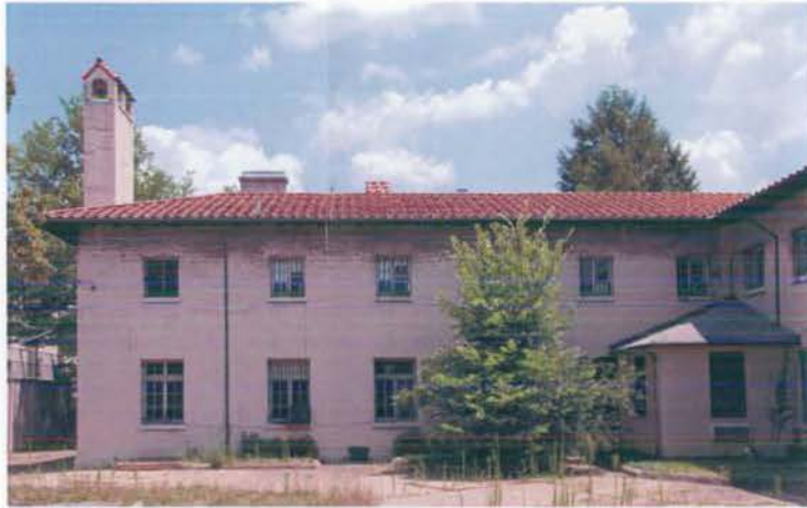
EXISTING CHANCERY WING ROOF
