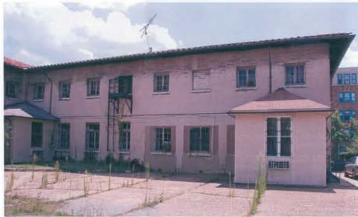
EXISTING CHANCERY WING WINDOWS
