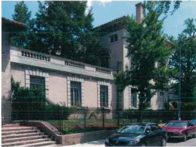
VIEW OF TERRACES AT EXISTING COURTYARD
