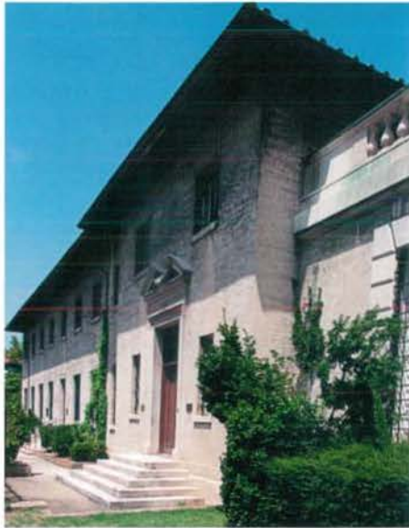
VIEW OF EXISTING CHANCERY
