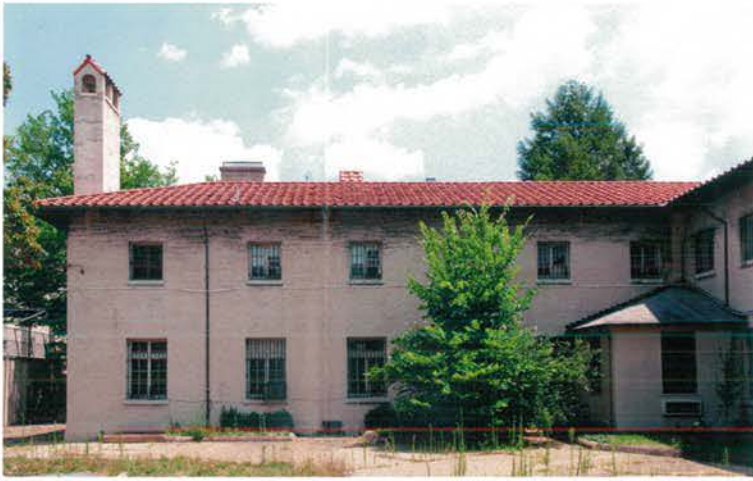
EXISTING CHANCERY WING ROOF
