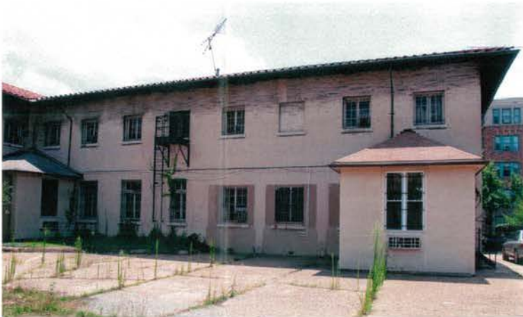
EXISTING CHANCERY WING WINDOWS
