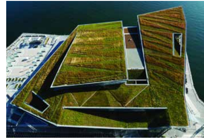
1 EXTENSIVE GREEN ROOF
