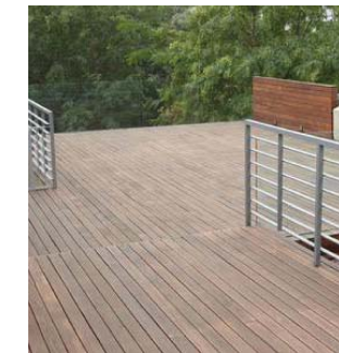
3 Wood Decking on Pedestal System
