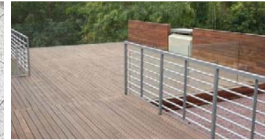
2 Wood Decking on Pedestal System
