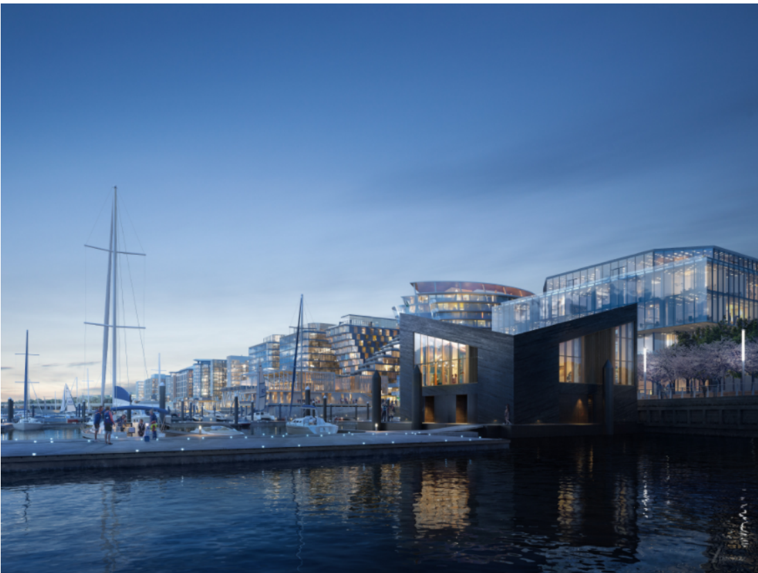
Water Building 3: View North
