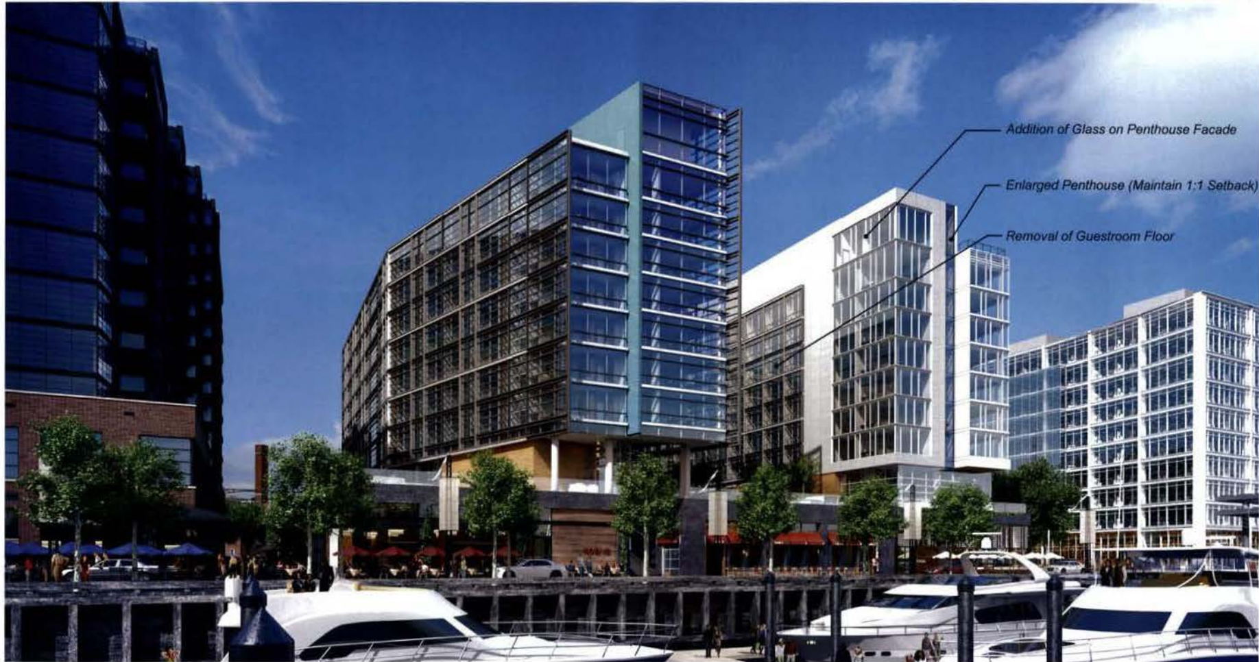
A) Interior Space and Square Footage Adjustments within the Building Envelope B) Penthouse Changes on Rooftop
