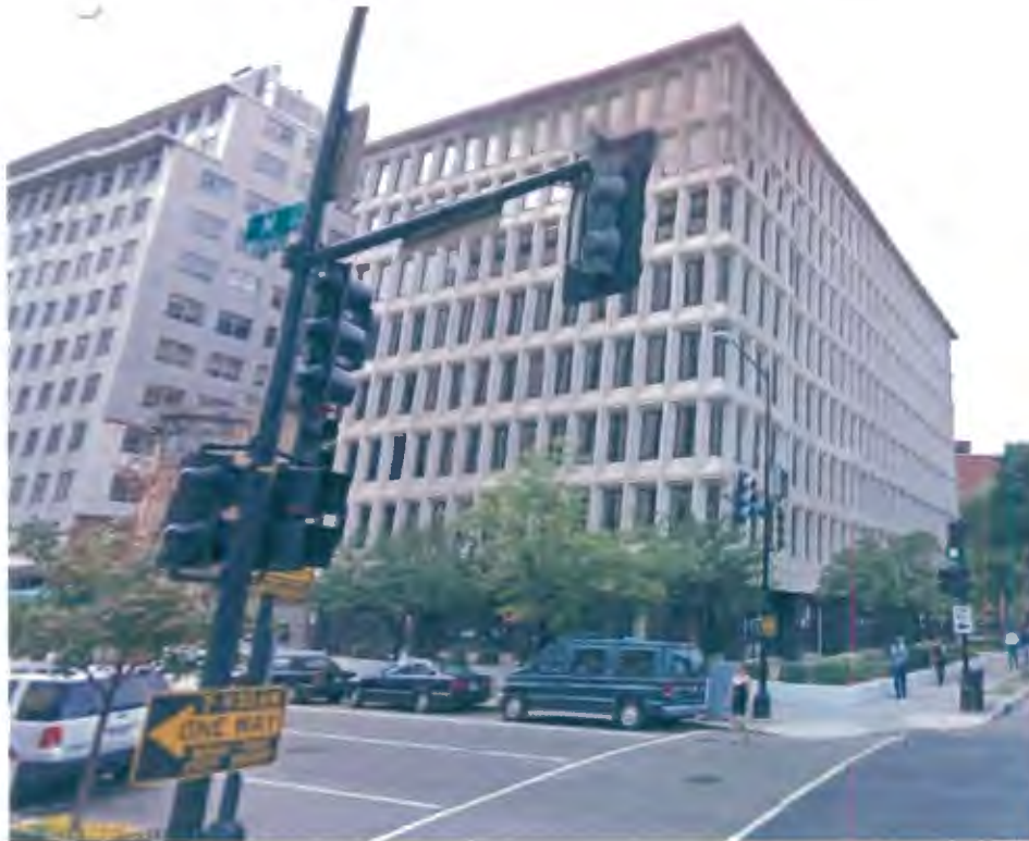
Subject Property viewed from the south 1730 Rhode Island Avenue (130 feet) on the left
