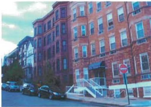
3. View looking North, directly across from the site
