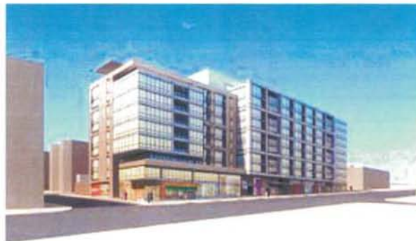
4. New Development - 14th Street Facade - View looking West
