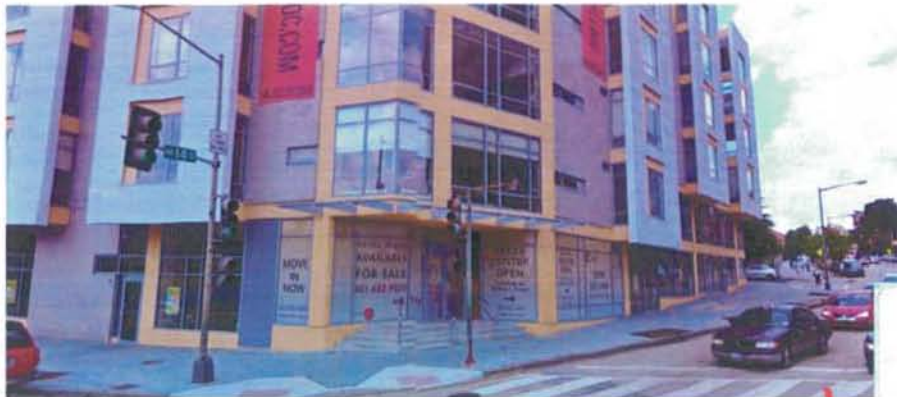
2. NEW DEVELOPMENT "SOLEA", CORNER OF 14TH ST & FLORIDA AVE, NW
