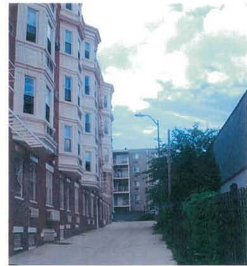
2. View looking North down public alley directly across from the site
