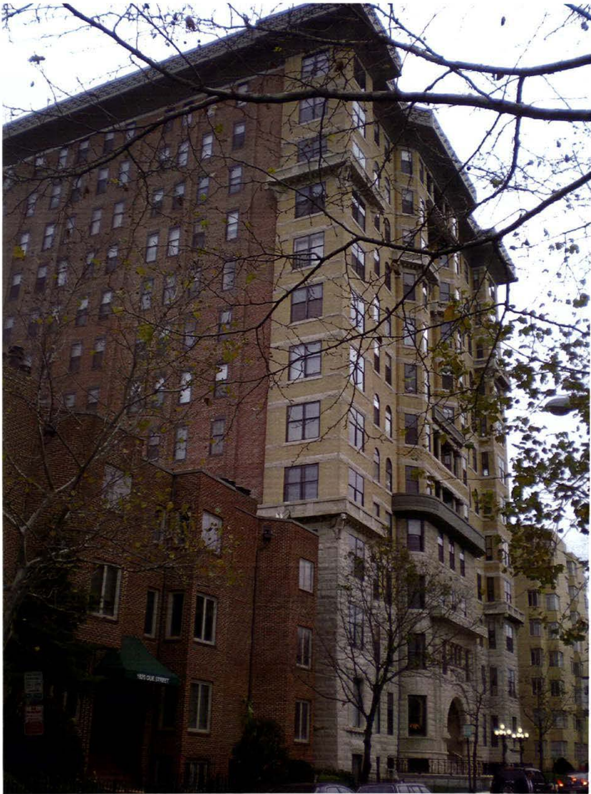
View of 1615 Q Street (the Cairo) on the north side of Q Street just east of the subject site
