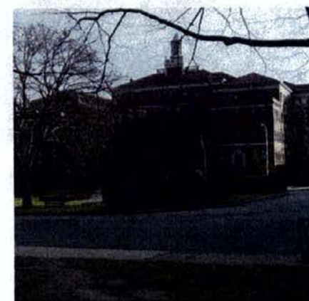
Top: CT Buildings
