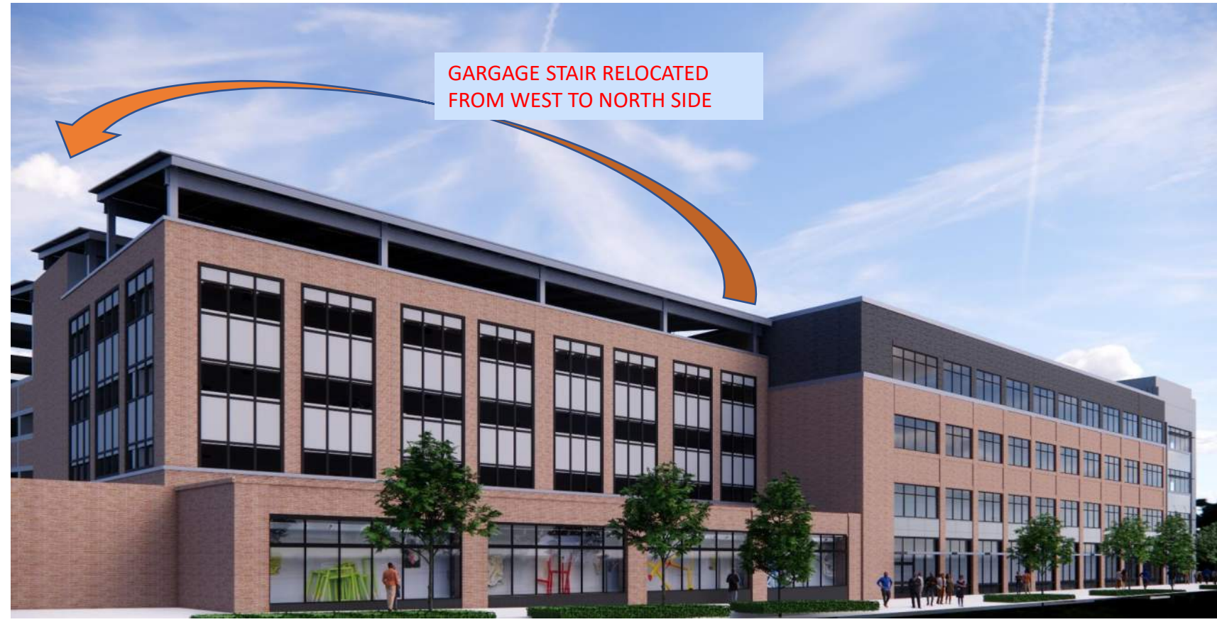
A - VIEW ALONG NAYLOR ROAD
