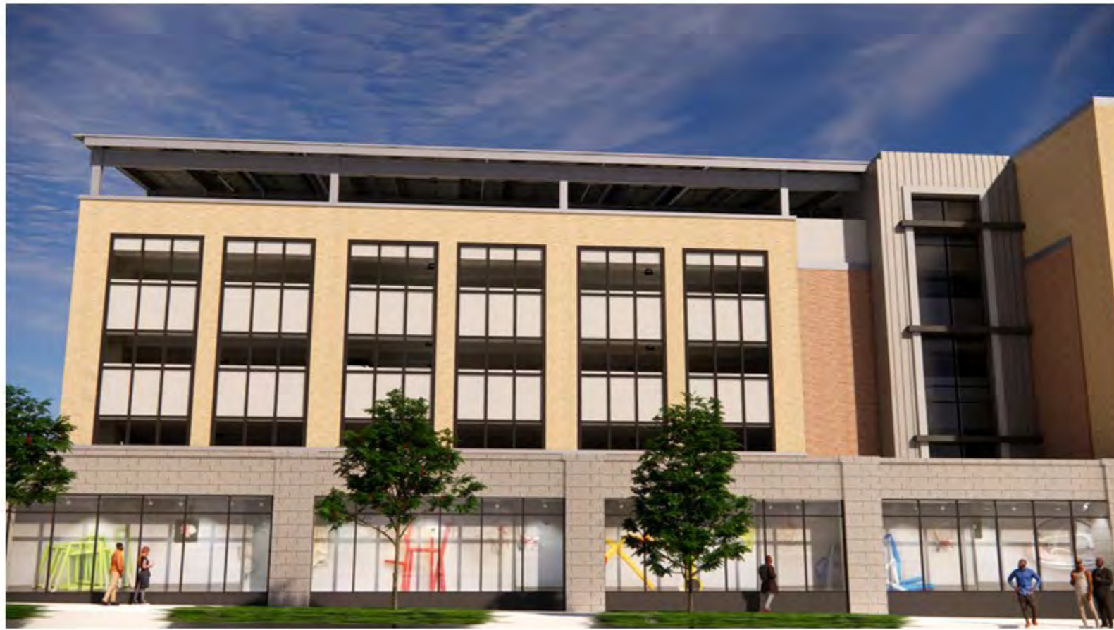
A - VIEW FROM ACROSS NAYLOR ROAD
