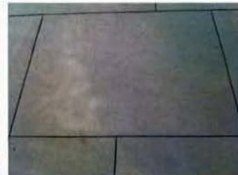
Staggered Saw-Cut Joints
