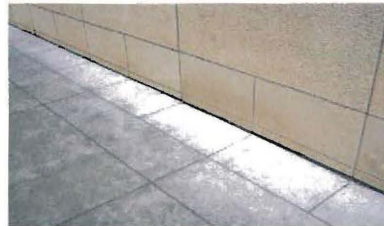
Saw-cut Concrete
