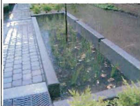
6. Residential Rain Gardens
