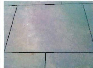
Staggered Saw-Cut Joints
