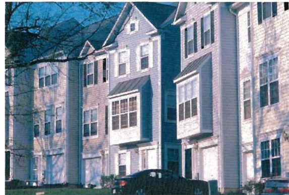
The Townhomes at Oxon Creek
