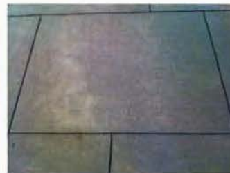
Staggered Saw-Cut Joints
