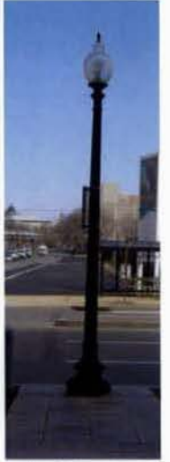
Typical Street Light
