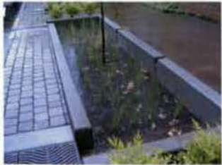
6. Residential Rain Gardens
