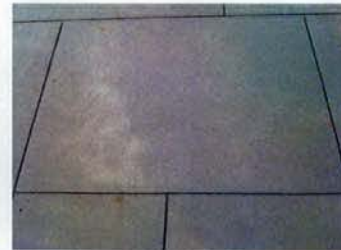
Staggered Saw-Cut Joints
